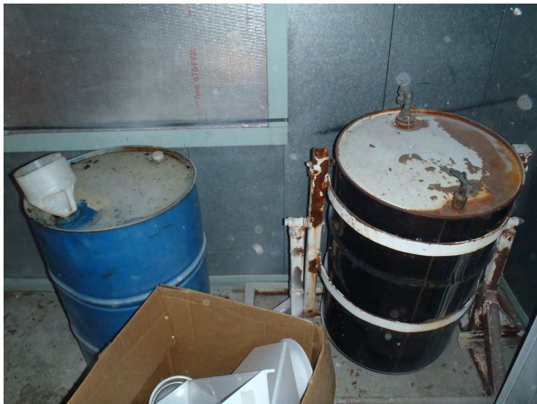
Photo 32: Waste drum inside paint booth
