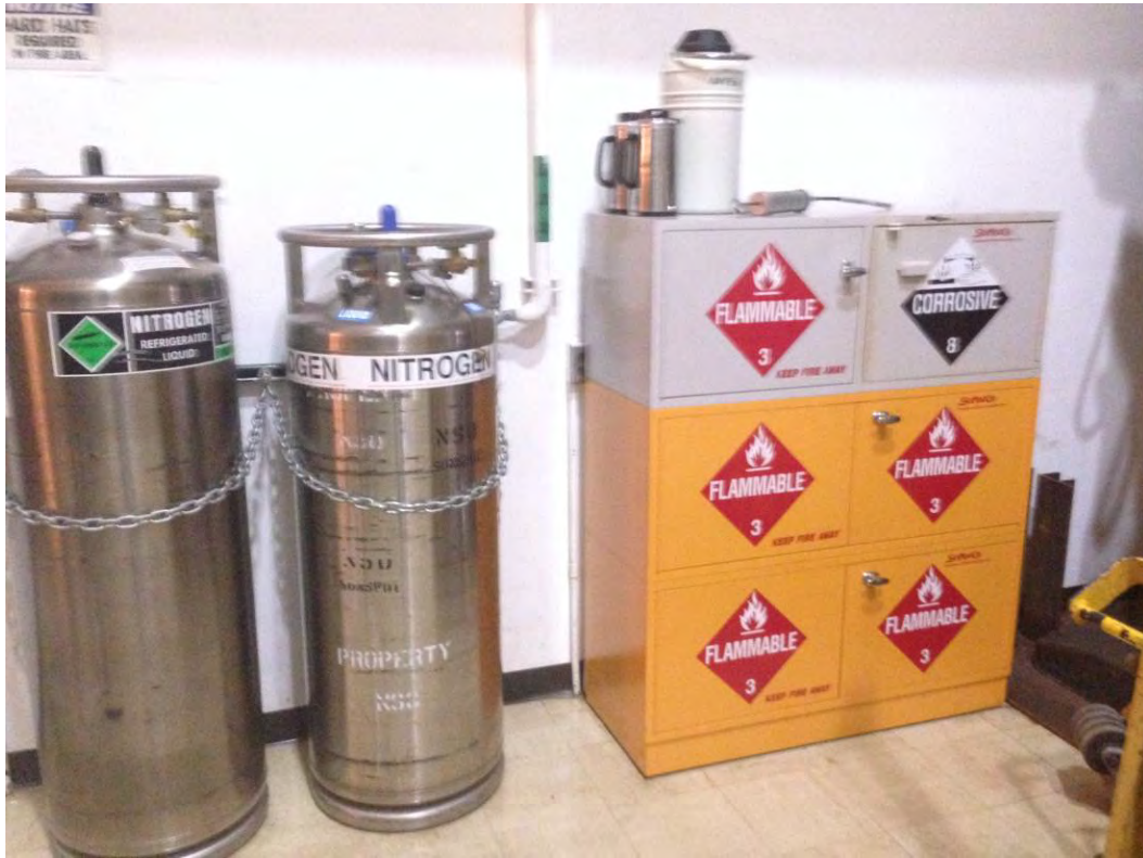
Photo 49: Flammable lockers and nitrogen tanks inside Dunn Solar Telescope
