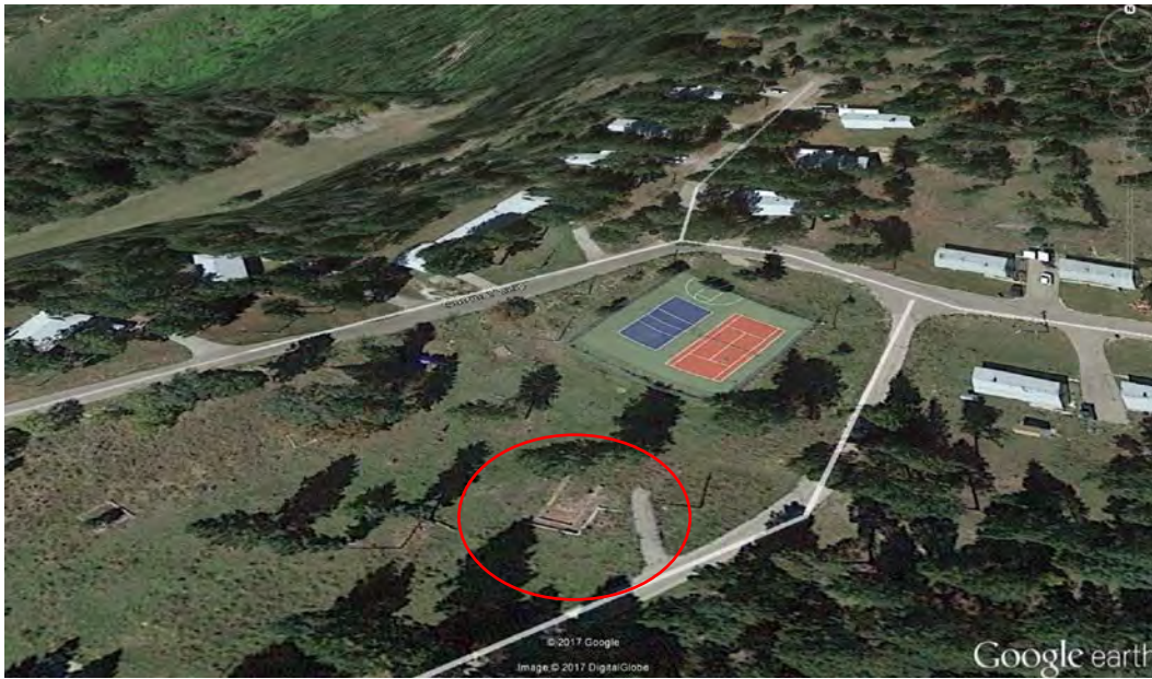
Photo 12. Red circle identifies the location of former Building 2028's foundation, just south of the recreation court
