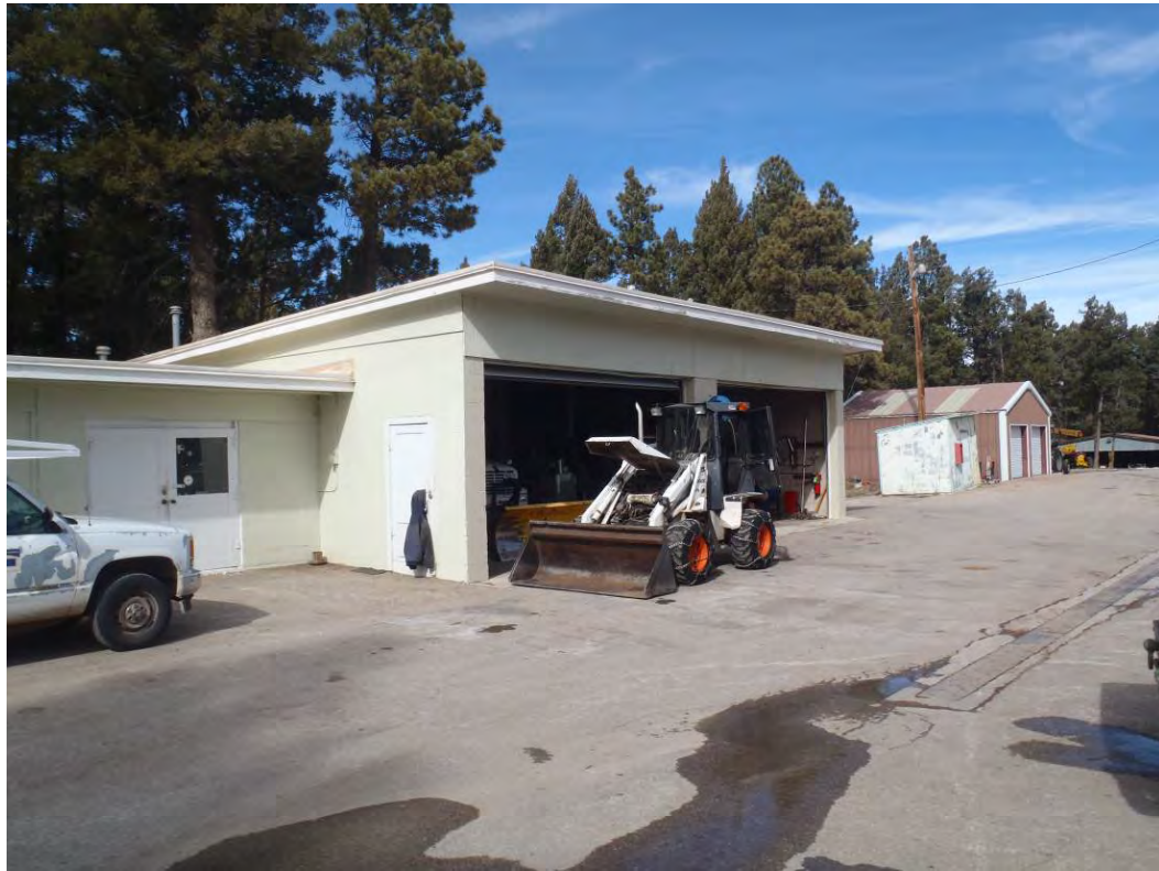
Photo 27: Maintenance garage facing northwest
