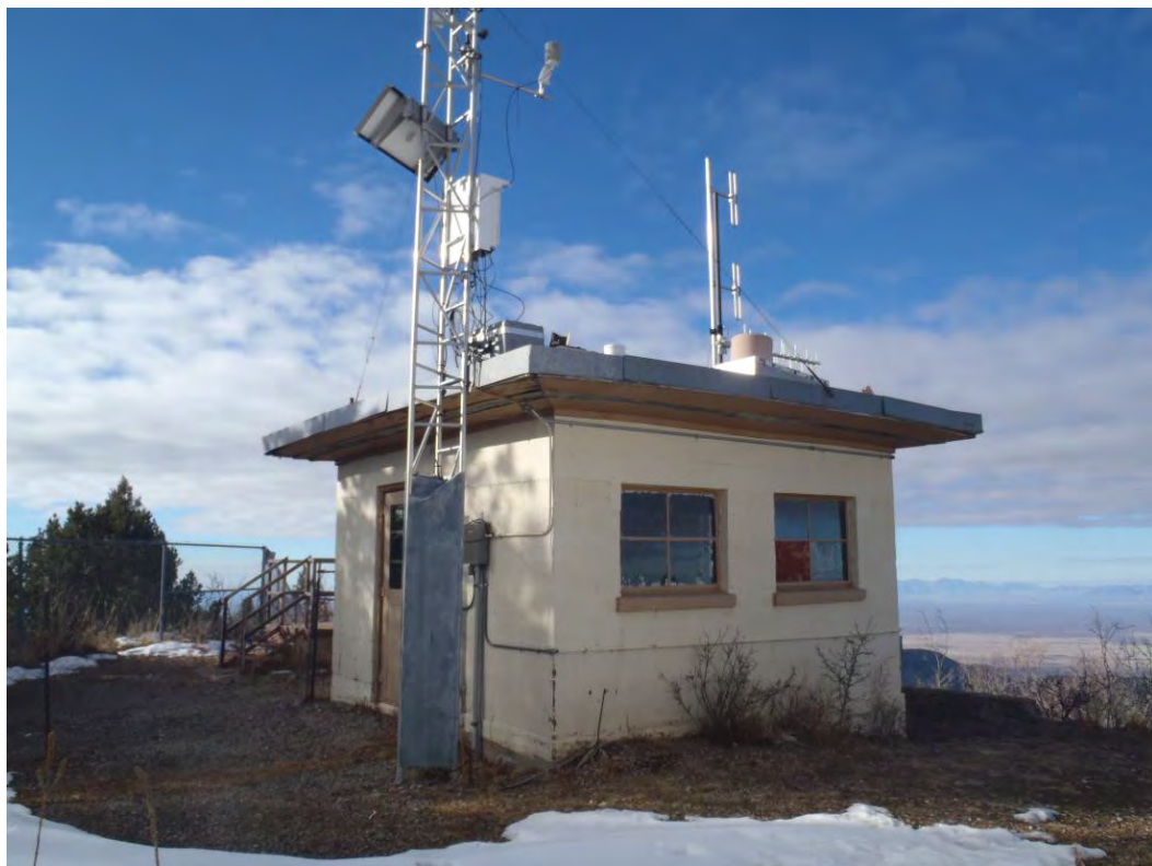
Photo 54: Weather station facing west
