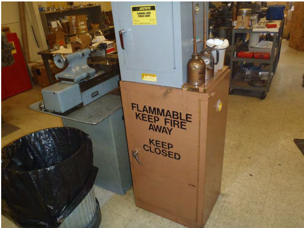
Photo 36: Flammable locker inside main lab
