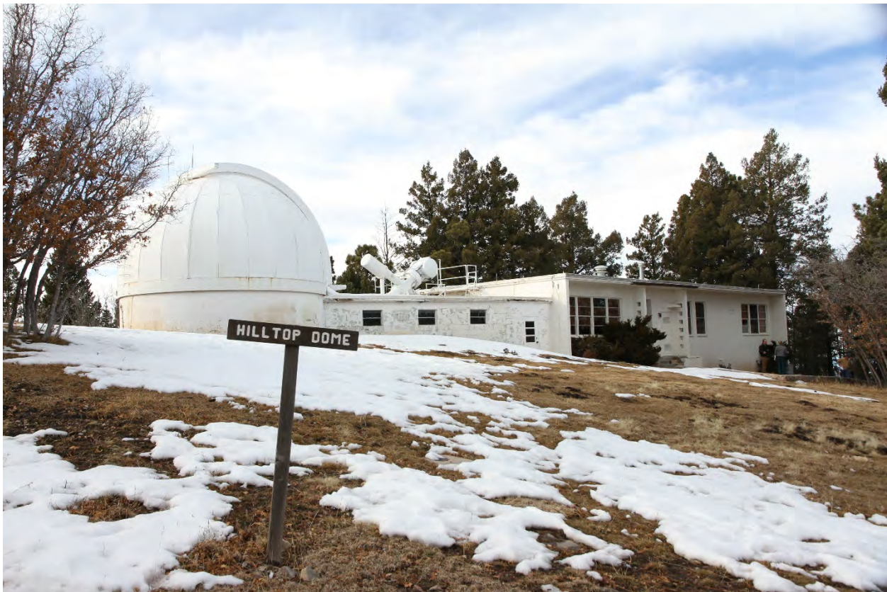
Photo 5. The Hilltop Laboratory (right) with the Patrol Dome (left), connected by a corridor addition
