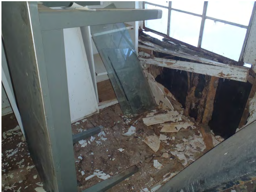
Photo 70: Inside Quonset hut near residential area
