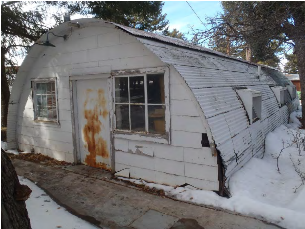
Photo 67: Storage Quonset hut
