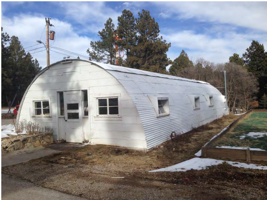
Photo 64: Quonset hut near administration building facing northeast
