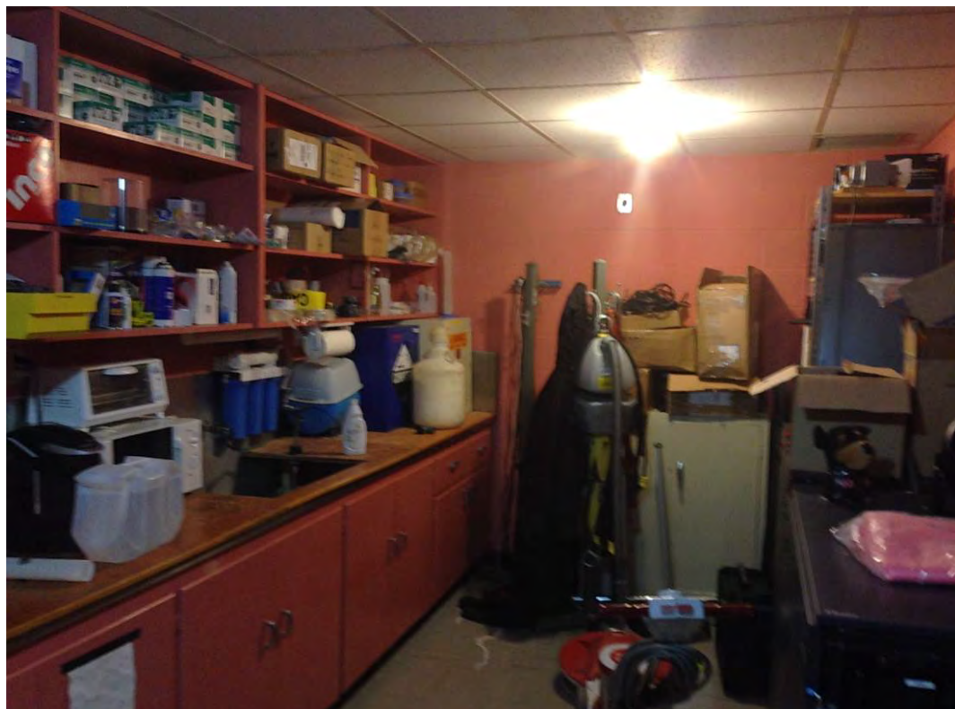
Photo 52: Flammable and corrosive lockers at Dunn Telescope building
