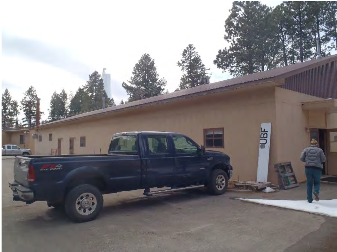
Photo 18: Machine shop facing south
