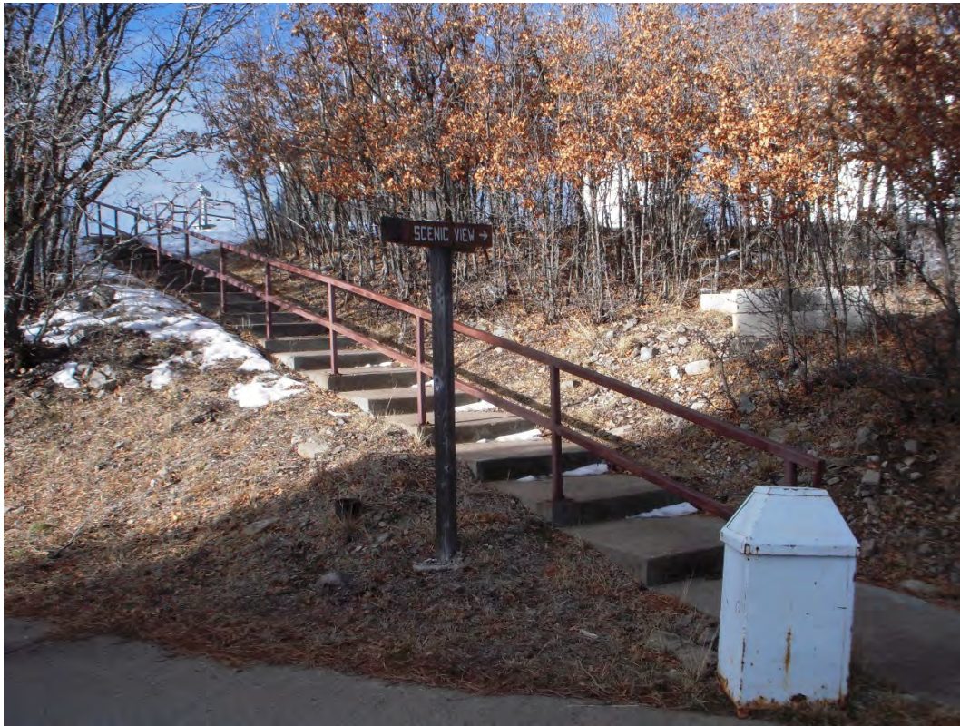
Photo 11. Outdoor stairwell near the DST
