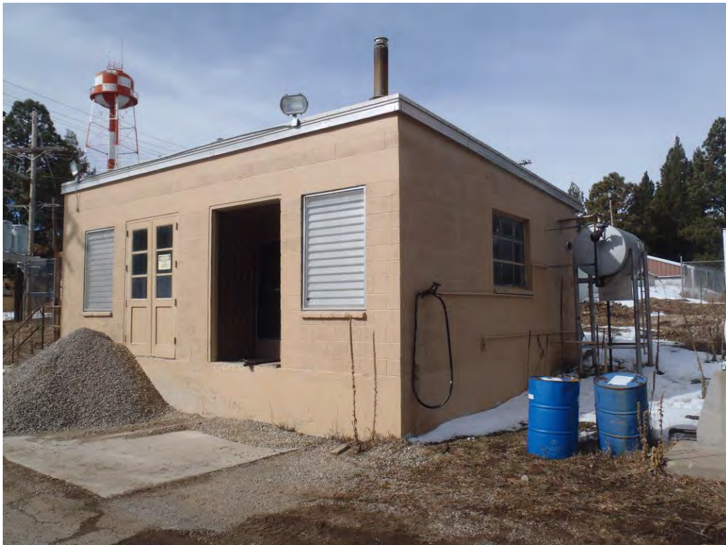
Photo 12: Backup generator building facing west
