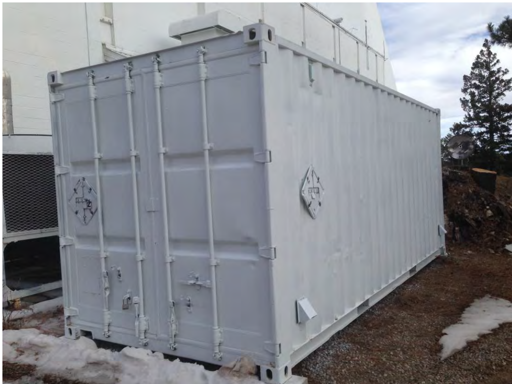
Photo 58: Mercury storage building facing south
