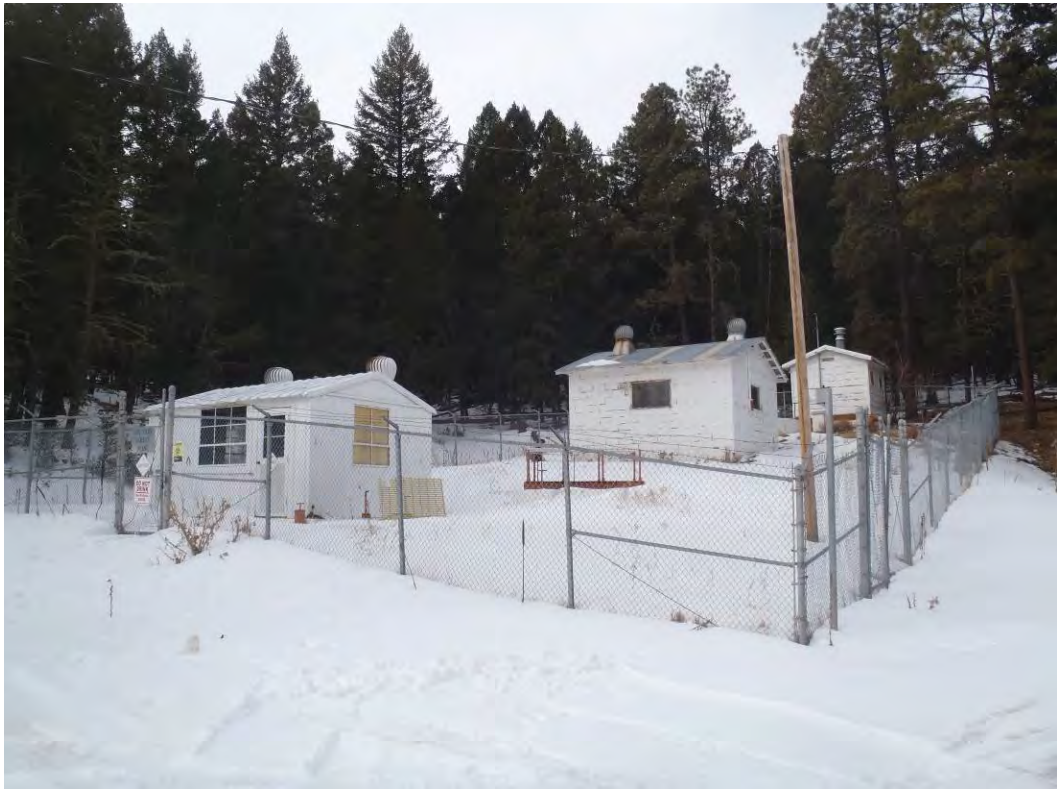
Photo 3: Wastewater treatment facility facing west
