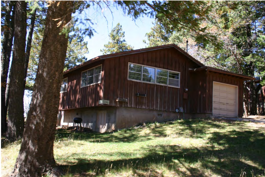
Photo 4. Building 3045, Redwood Family Housing on Hound Dog Hill
