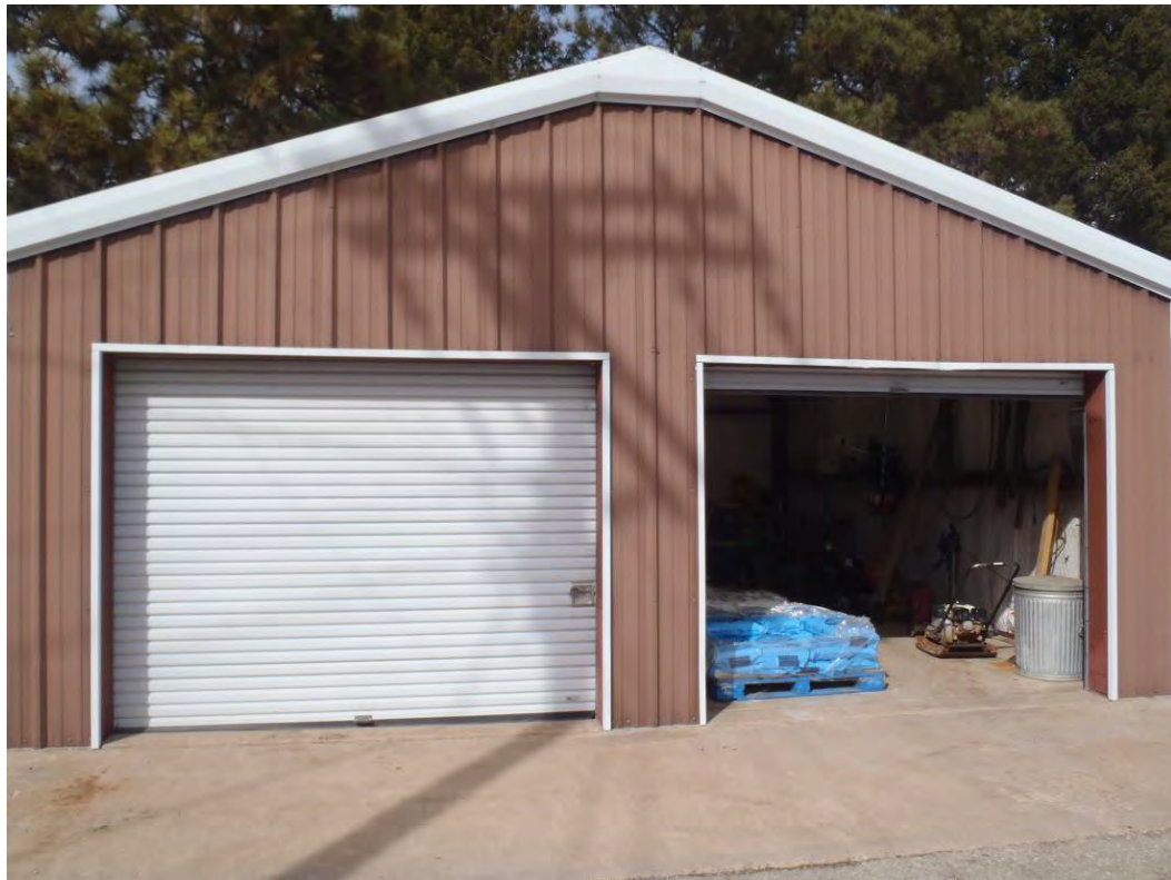
Photo 24: Hazardous waste storage building (left bay) and ground maintenance (right bay)
