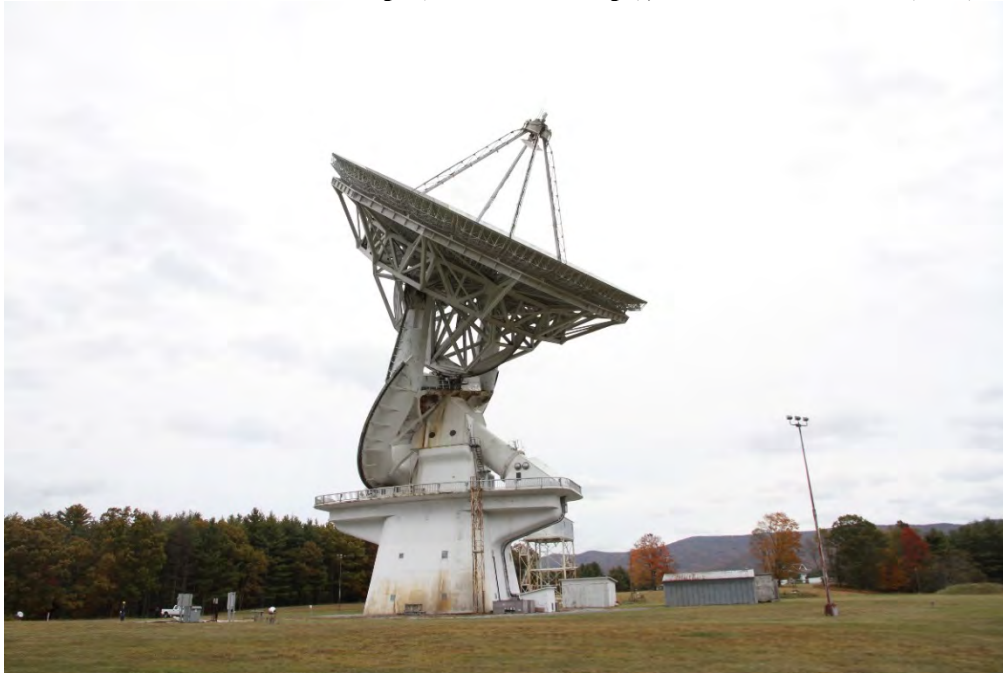
FIGURE 3.3-4 West side of the 43-meter Telescope (140-foot Telescope); view to the northeast (2014).
