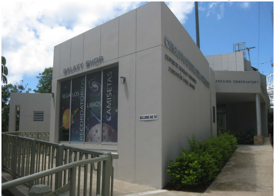
Photograph 5. Building #54 (NRHP Buildings #5), Visitor Center North elevation, view to the south.
