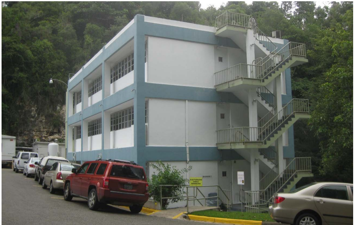
Photograph 4. Building #2, Administration Building Southeast corner, view northwest.
