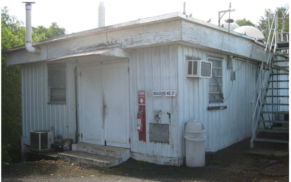
Photograph 8. Building #27 (NRHP Building #7), Photometry Shack/Optical Lab Northwest corner, view to the southeast.
