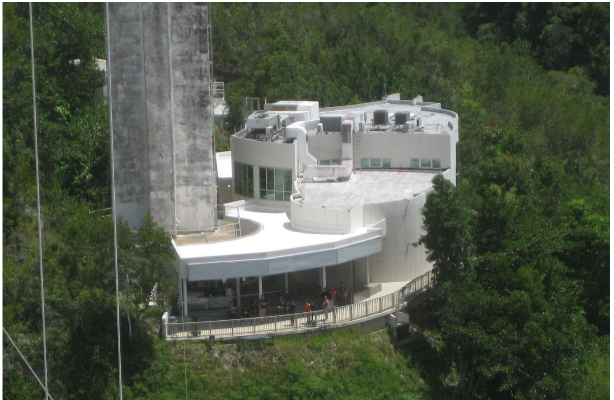
Photograph 6. Building #54 (NRHP Building #5), Visitor Center 2015 rear (south) addition, view to the north.
