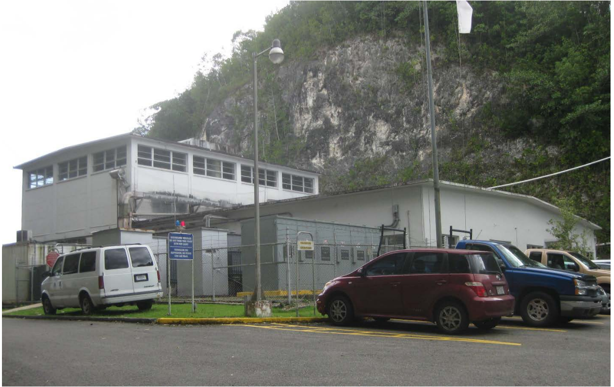
Photograph 2. Building #1 (NRHP Building #1), Operations Building Northeast corner, view southwest
