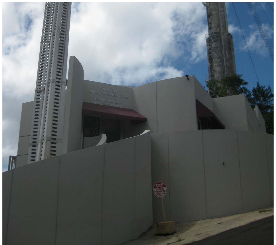
Photograph 7. Building #61 (NRHP Building #6), Learning Center South elevation, view to the north.
