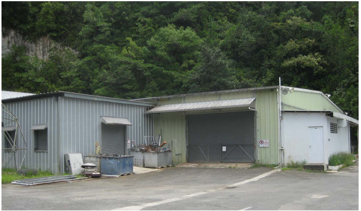
Photograph 10. Building #12 (NRHP Building #13), Maintenance Building Northeast corner, view to the southwest.
