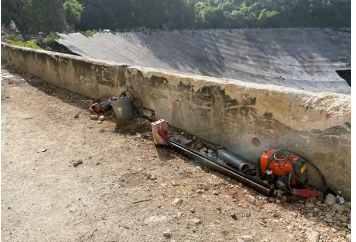
William E. Gordon (305-meter) Radio Telescope – Rim Wall – 9 concrete cores taken from rim wall for testing. Cores are red circled areas.
