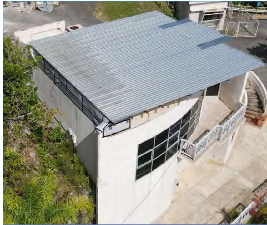
Learning Center (Building 61) After Temporary Weatherproofing, August 25, 2021
