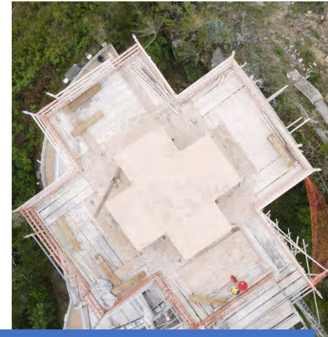
Tower 12 Waterproof Coating
