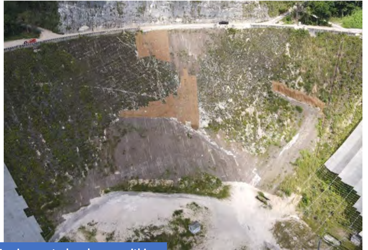
Erosion control underway within the Reflector Area
