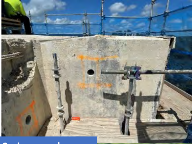
Tower 8 – Coring sample
