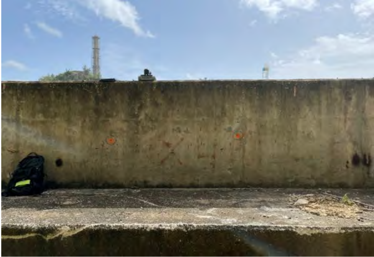
William E. Gordon (305-meter) Radio Telescope – Rim Wall – 9 concrete cores taken from rim wall for testing. Cores are red circled areas.
