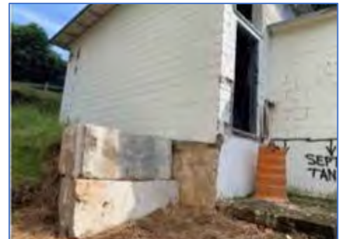
Cable Car Building (Building 5) Temporary Retaining Wall
