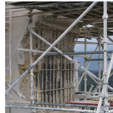
Tower 12 Repair Underway
