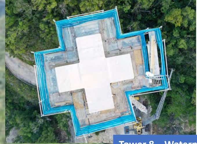
Tower 8 – Waterproof Coating
