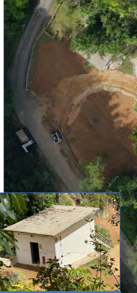
Cable Car Building (Building 5) During Clean-up
