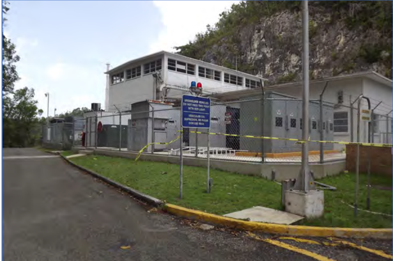
Operations Building (Building 1) Before
