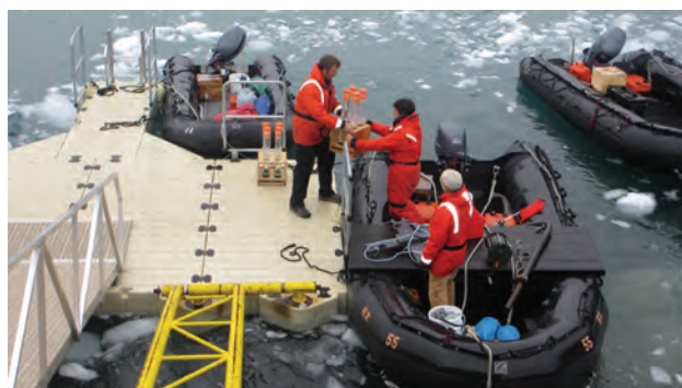
A new floating dock and ramp system at Palmer Station provides improved safety and efficiency for conducting small boating operations in support of marine research. Credit: Rebecca Shoop and Bob Farrell, Antarctic Support Contract
