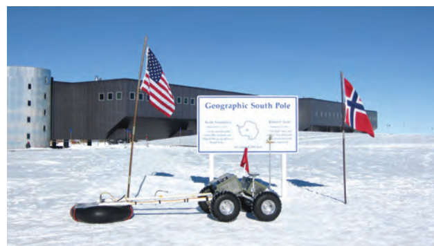
The Yeti robot (pictured in the foreground) was used successfully last season to remotely locate sub-surface areas with buried structures or voids so that the overlying snow could be made safe for surface activities. Credit: James Lever, U.S. Army's Cold Regions Research and Engineering Laboratory
