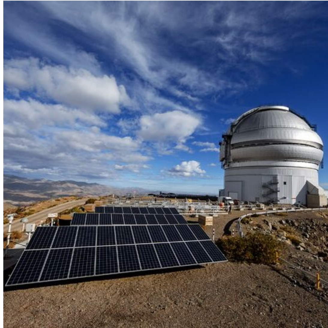
Gemini-S Observatory photovoltaic panels
